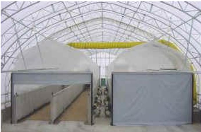
*Composting facilities as shown on this picture can transform several hundreds of tonnes of organic waste into high-quality compost in a short period of time without negatively impacting the environment.*
