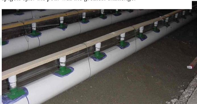
*Figure 3. In 2003, we used a 1” x 2” section of wood on top of the spigots allows the aeration holes to be recessed and allows easier leveling of the concrete floor.*
