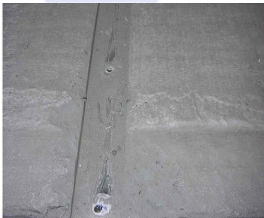
*Figure 2. Concrete floor with 3/4” deep trench protects the aeration piping.*
