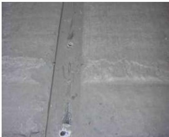
Figure 3. Concrete floor with 3/4” deep trench protects the aeration piping.
