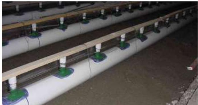
Figure 2. In 2003, we used a 1” x 2” section of wood on top of the spigots allows the aeration holes to be recessed and allows easier leveling of the concrete floor.
