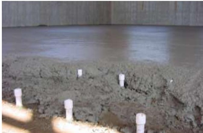
Figure 1. Pouring concrete for an aerated floor in 2002. Finding the spigots after the pour was the greatest challenge!
