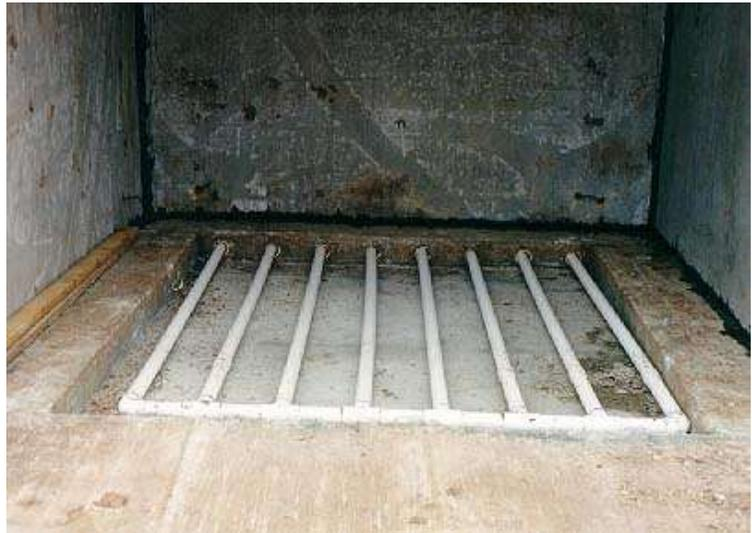
*Figure 4. One of our first aerated floor designs that allowed the loader wheels to ride along the footings for the wall.*
