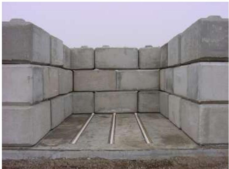
*Figure 5. A 2" PVC pipe in a 3.5 x 3.5 inch trench in the concrete allows the loader to drive on the floor without damaging the piping.*
