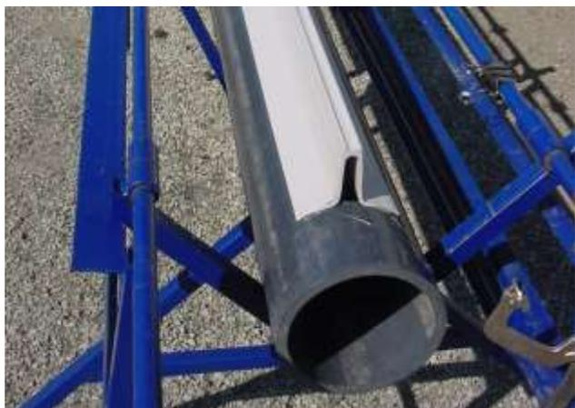
Figure 8. Installing the PVC extrusion onto the HDPE pipe to be completely embedded in the concrete floor.
